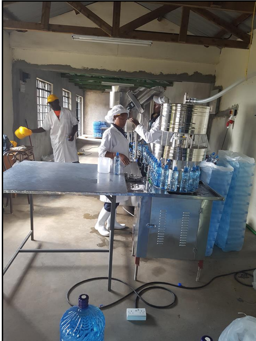
The newly installed semi-automatic water processing machine in operation
